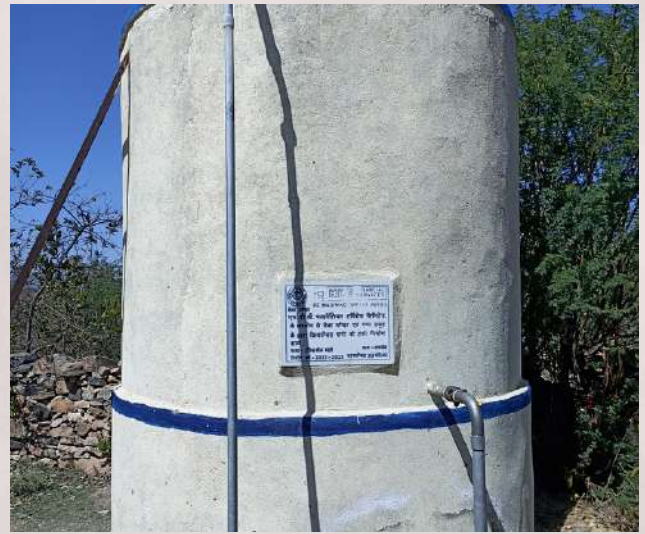
Fig 9: Water storage tank at Sakroda village.
