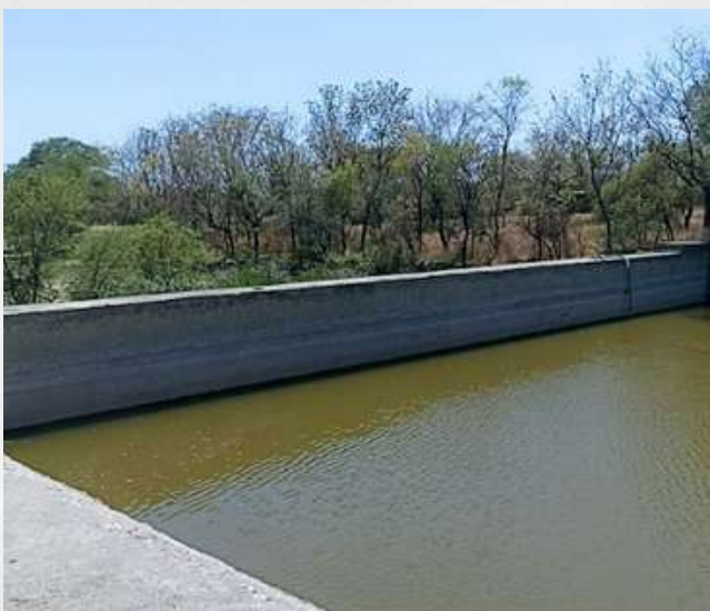
Fig 3: Check dam at Sakroda village.
