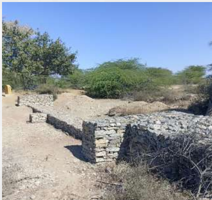
Fig 1: Gabion structure preventing soil erosion.
